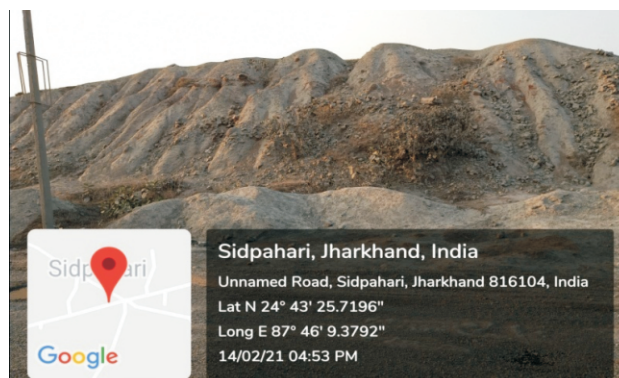
Removal of Top Soil, for mining at Sidpahari
